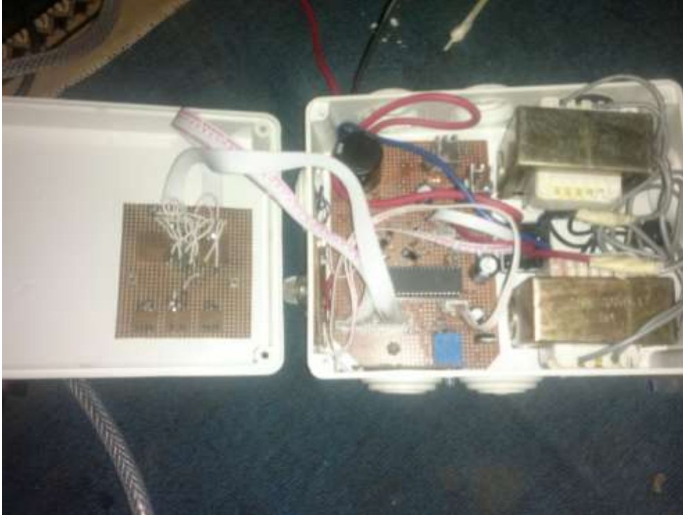
Figure 4.2: Constructed automatic fire control system
